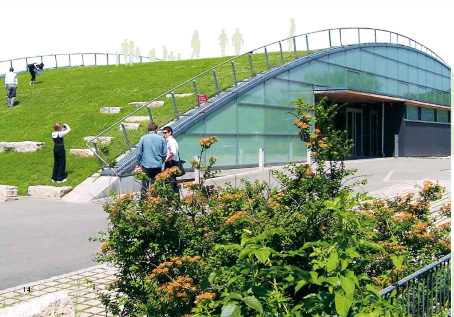
Once the Floratherm® elements were installed approx. 0,15 m of intensive substrate was blown onto the area.
