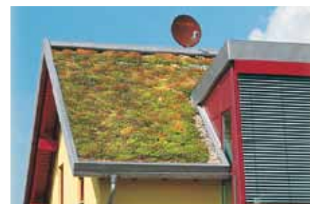
With this roof, which has a pitch of approx. 30°, a shear barrier was installed within the roof area, in addition to the stable eaves upstand.
